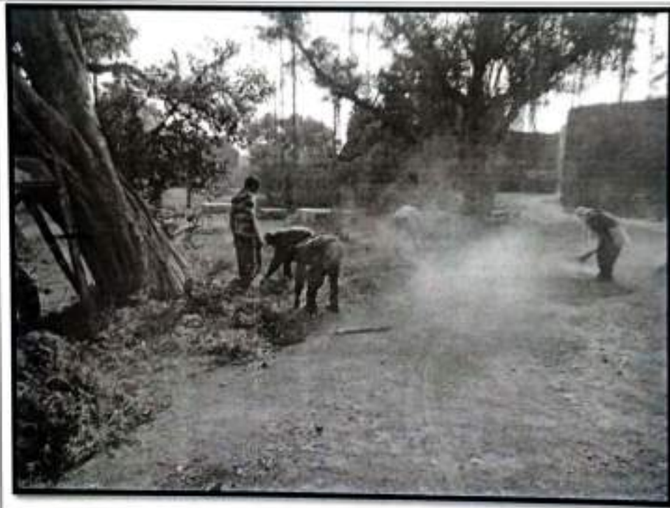
NSS Unit Ashvi Kd. conducted road repairing
