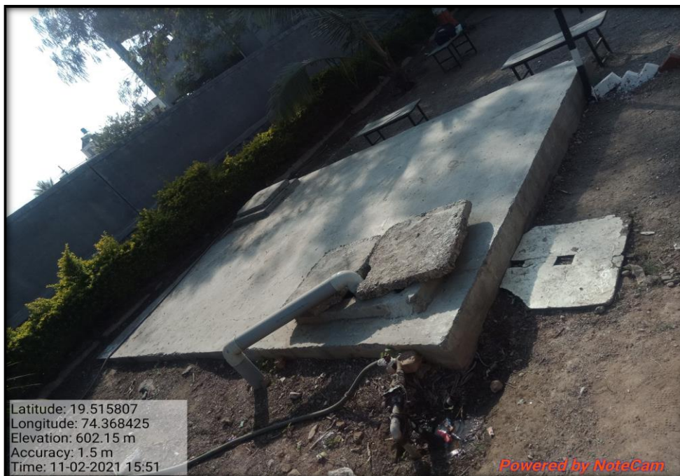
Tank constructed for Water Collection
