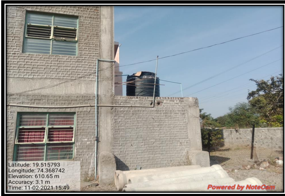
Maintenance of water and effective Water distribution System
