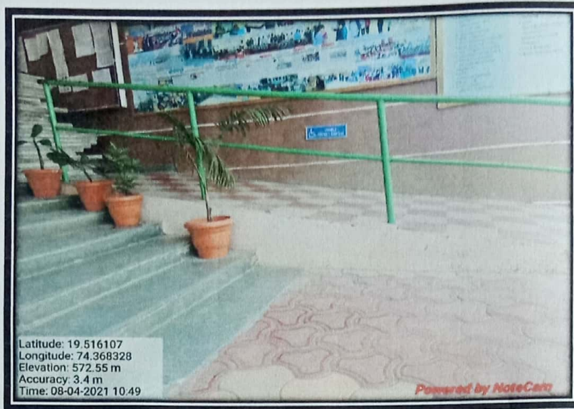
Actual photograph for the Ramp facility in the institution
