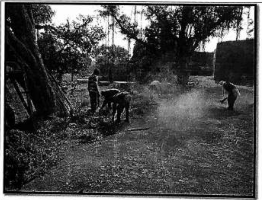
NSS Unit Ashvi Kd. conducted road repairing
