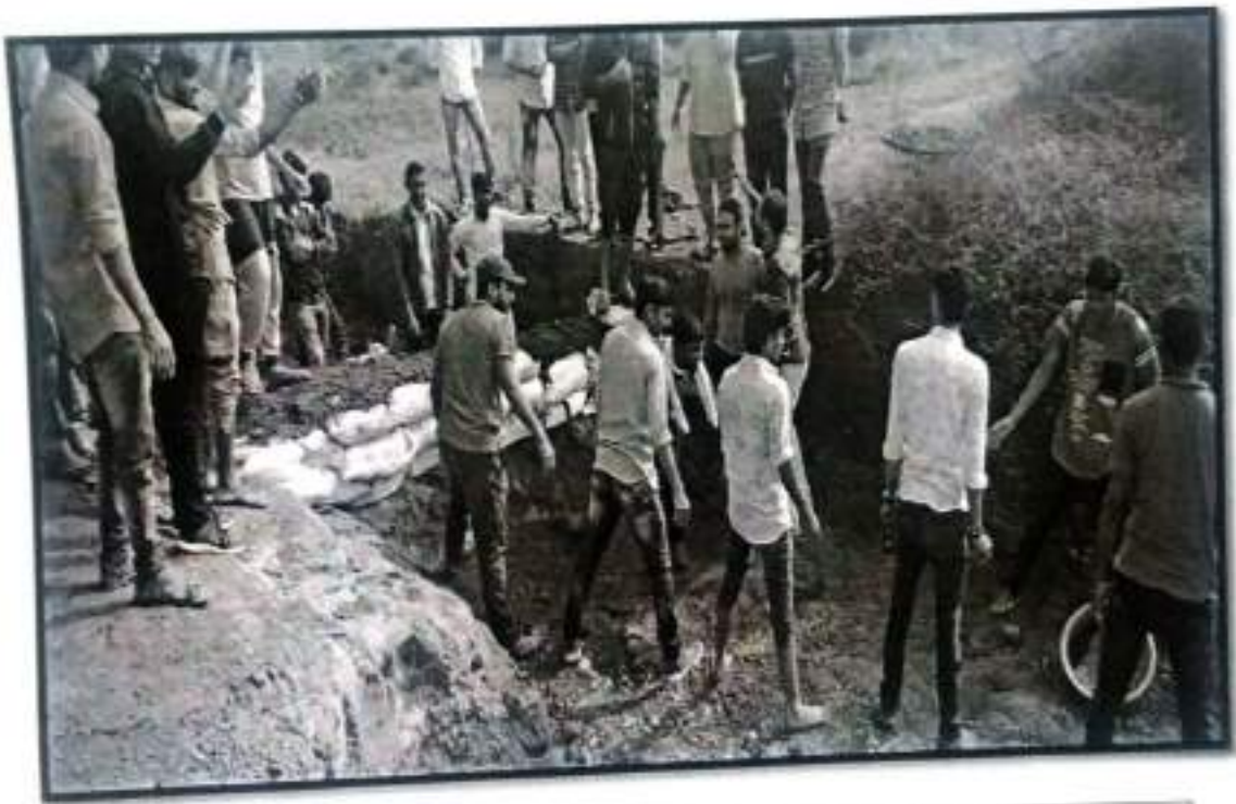
N.S.S Camp Volunteers Made Check dam in Pratappur.
