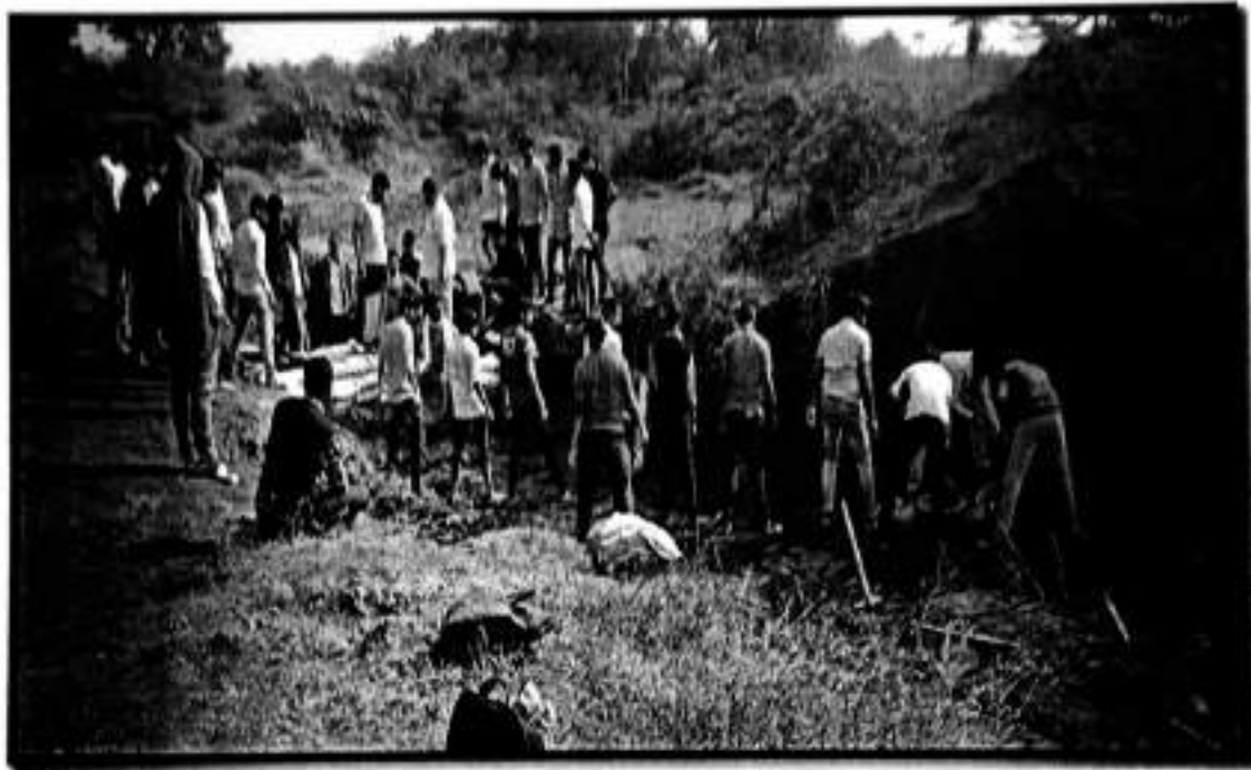
N.S.S.Camp Volunteers during Check dam At -Pratappur
